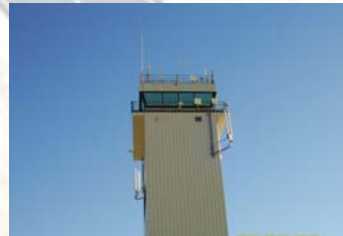
New ADS-B Antennas on Tower
